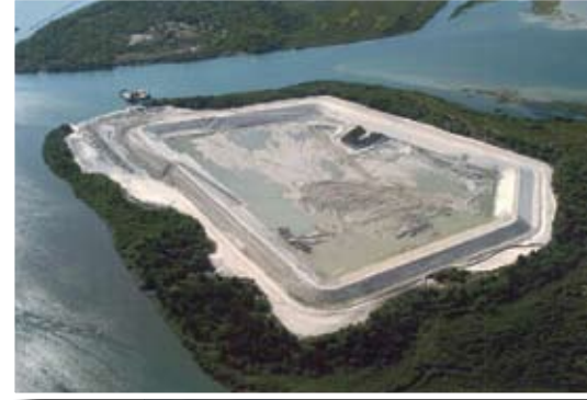
MSA 434, one of 54 Dredged Material Management Areas (DMMAs) located along Florida's east coast, provides space to dewater and store material dredged from the Atlantic Intracoastal Waterway (ICWW) navigation channel.
