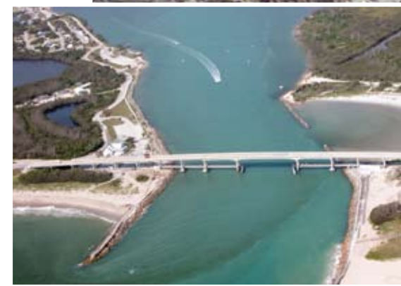
Sebastian Inlet dredged channel design provides safe navigation through the flood shoal to the ICWW. Photo courtesy of St. Johns River Water Management District.
